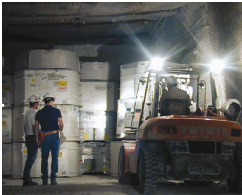
Waste being stacked in a disposal vault at the Waste Isolation Plant (WIPP) in New Mexico USA (courtesy WIPP information centre)
