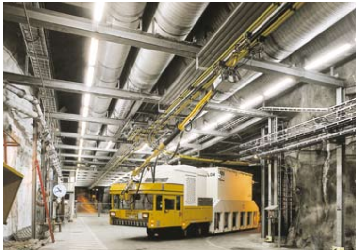
Underground transport facilities at a disposal facility in Sweden (courtesy SKB)
